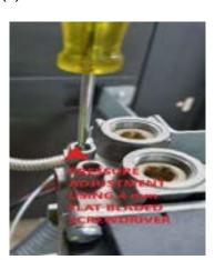
The pressure test points for the inlet and outlet (burner) pressure measurements are located at the top of the gas valve casing.
