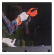
Step 3: With one hand holding the glass pad, with an upward motion lift the top of the glass until engaging with the top of the inner fascia. Thebottom of the glass is now clear of the bottom supporting channel. Swing the bottom of the glass outward with one handholding the glass pad andtheotherhandgrippingthebottomcentreedgeof the glass.
