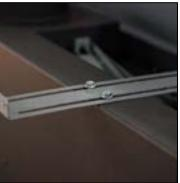
The rear stand-off spacers maintain a clearance of 250 mm from combustible materials. The sidestand-off spacers maintain a clearance of 250 mm from combustible materials.
